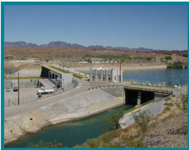
Headgate Rock Dam, Colorado River.
