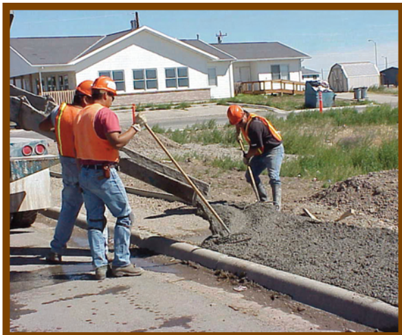
Construction crew pouring concrete sidewalk.
