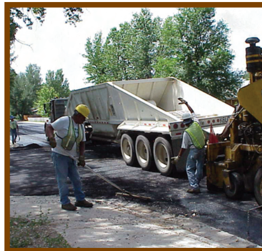
Road construction crew at work repairing street.
